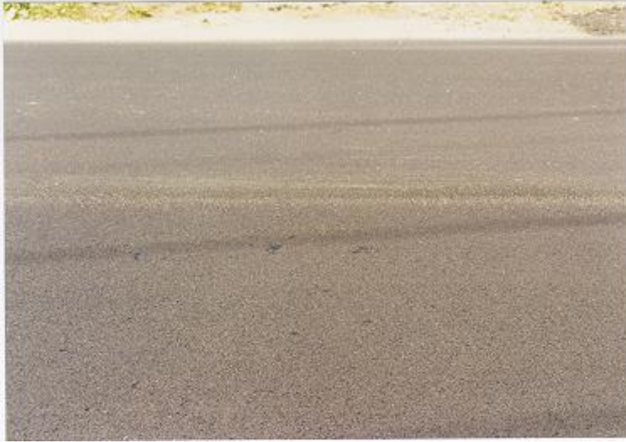
Photo 13. Erie County S.R. 4022 Rolled Wearing Course with Shingles
