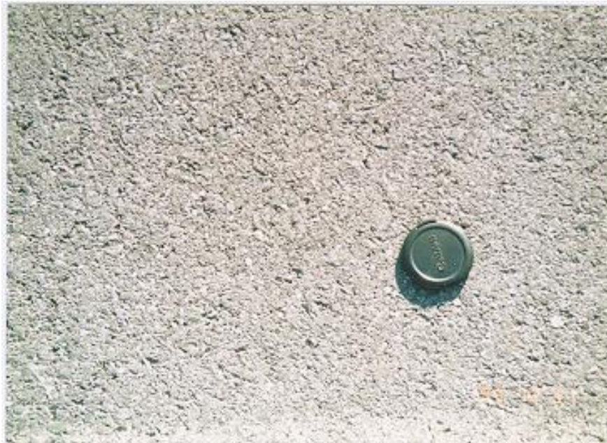
Photo 3. Lehigh County, Saucon Valley Road Close-up view of the bituminous concrete with fiberglass asphalt shingles in ID-2 wearing course at Sta 36+90 in 1994.
