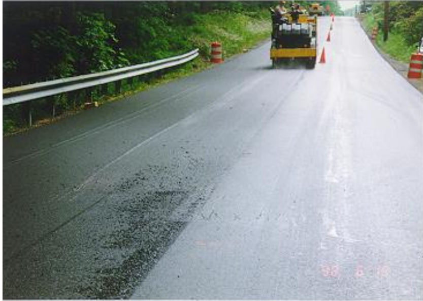
Photo 11. Dauphin County S.R. 325 Shingle Material Picked Up By Roller
