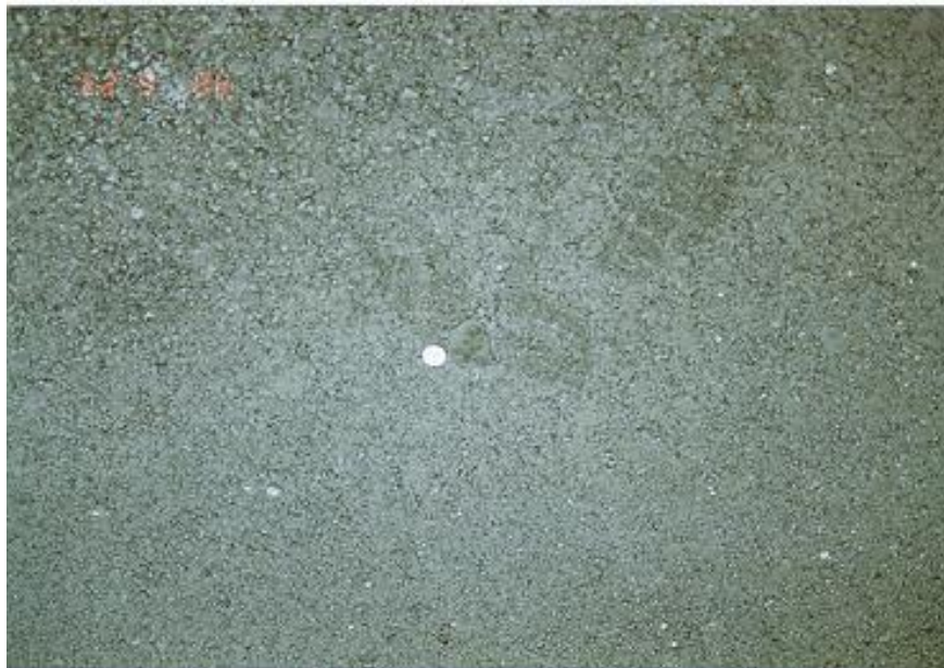
Photo 10. Dauphin County S.R. 325 Compacted Wearing Course with Shingles
